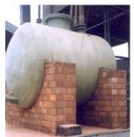
Figure 8. Tank foundation with acid resistant bricks<sup>xvii</sup>
