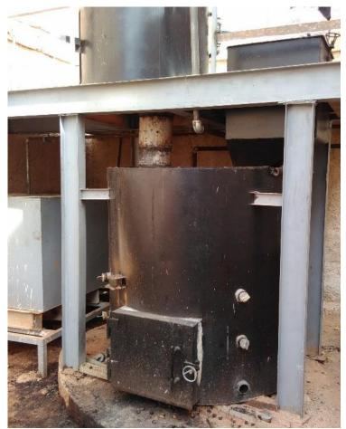
Figure 5. H2CP pyrolizer installed under a vertical boiler in a cottonseed oil factory in Burkina Faso; pyrolizers can be used out of cashew processing units, thus generating fuel savings to neighboring industries
