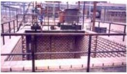
Figure 9. Brick lining of underground tank<sup>xviii</sup>
