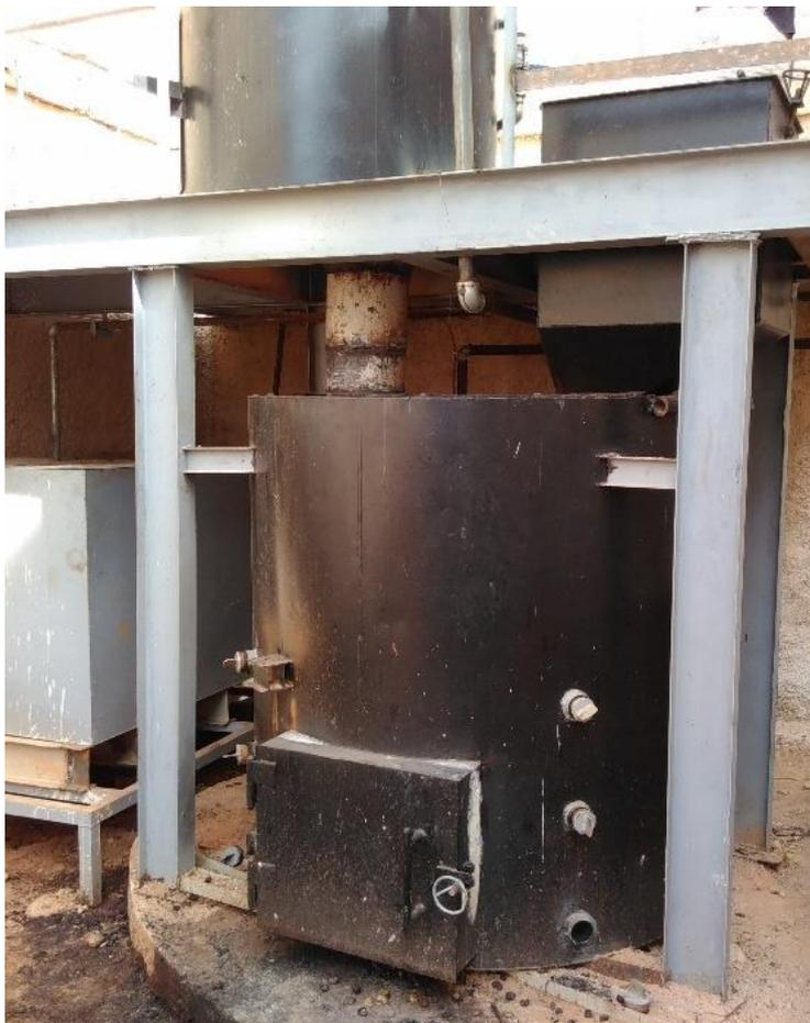
*Figure 5. H2CP pyrolizer installed under a vertical boiler in a cottonseed oil factory in Burkina Faso; pyrolizers can be used out of cashew processing units, thus generating fuel savings to neighboring industries*
