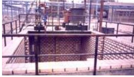
Figure 9. Brick lining of underground tank<sup>xviii</sup>
