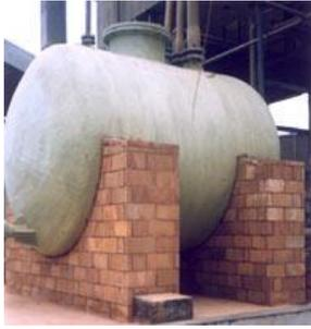
Figure 8. Tank foundation with acid resistant bricks<sup>xvii</sup>
