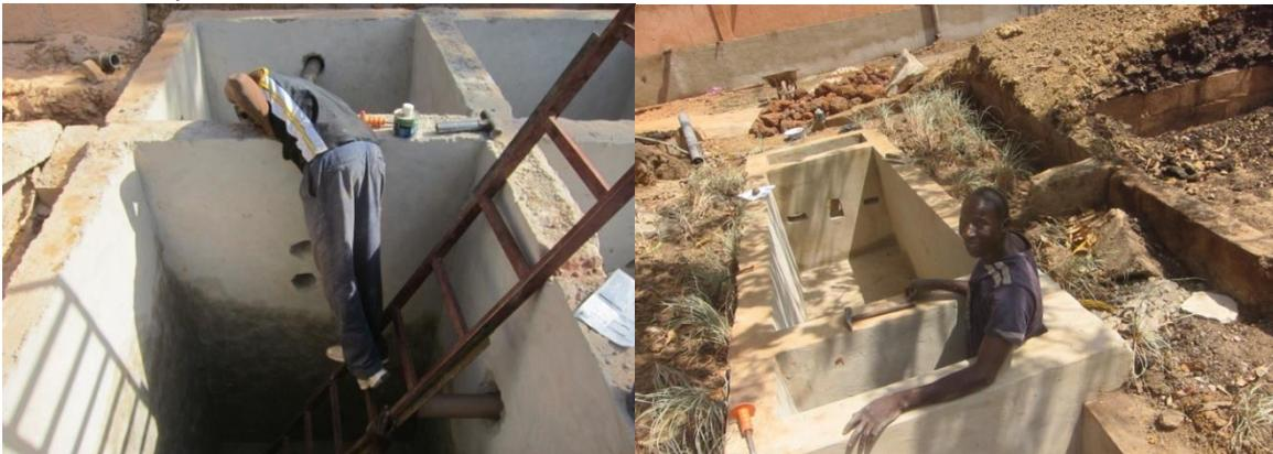
Figure 7. Construction of septic tanks for water treatment
