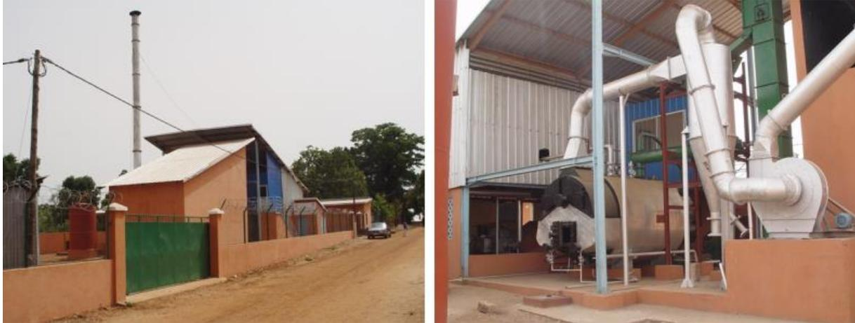
*Figure 12. Biomass power plant at Safim (left). Photo of the boiler (right)*
